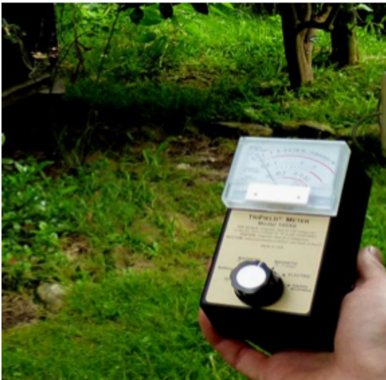
Fig.3 The meter registering zero EMF . Taken next to the Power transformer. Colours have been contrasted to show up dial.
